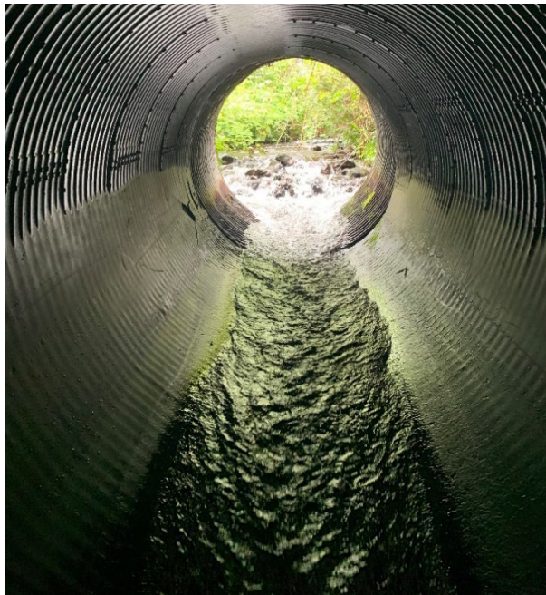
Figure 9.7-4: Insufficient water depth
