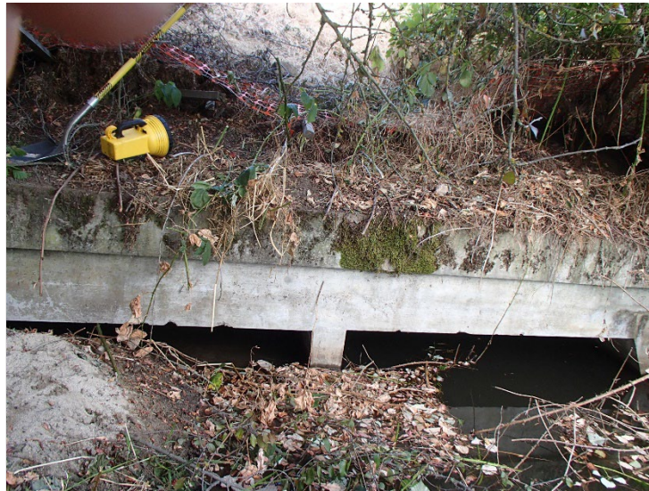
Figure 9.7-2: Inlet sediment accumulation
